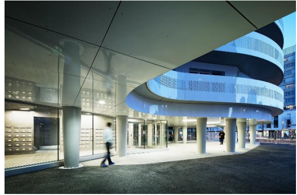
Fig. 5. Entrance zone in building New'R Tower, ZAC Euro Nantes (Nantes, France); authors: Hamonic + Masson & Associates (2017) © Takuji Shimmura
