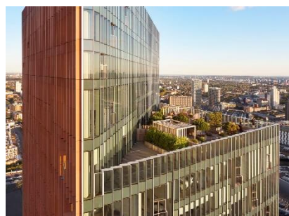
Fig. 8 Manhattan Loft Gardens (London, UK) – a common recreational terrace of the high-rise building for residents and their guests. Authors: SOM (2018). © Hufton + Crow.
