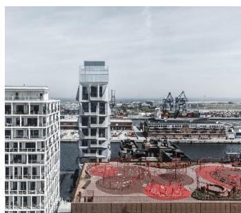
Fig. 7 The Silo (Copenhagen, Denmark), recreational areas with high-rise residential buildings and a revitalized port wharf. Author: COBE (2017). © Rasmus Hjortshøj – COAST
