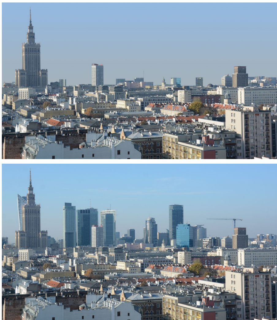
Fig. 4. Warsaw's cityscapes: end of 1980s (top) and 2015 (bottom). Source: author's materials
