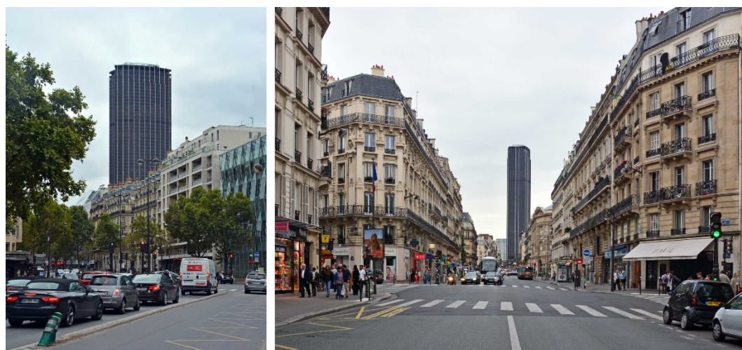
Fig. 2. Tour de Montparnasse in Paris (height: 210 m, completion: 1972, arch.: Beaudouin, Cassan, de Marien and Saubot) criticised for destroying the cityscape. Source: photograph by author
