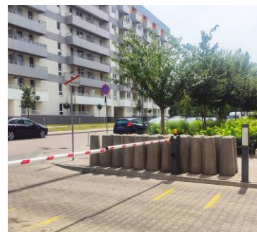
Fig. 7. Concrete bollards purchased by a housing association to fight against illegal parking. Source: by author
