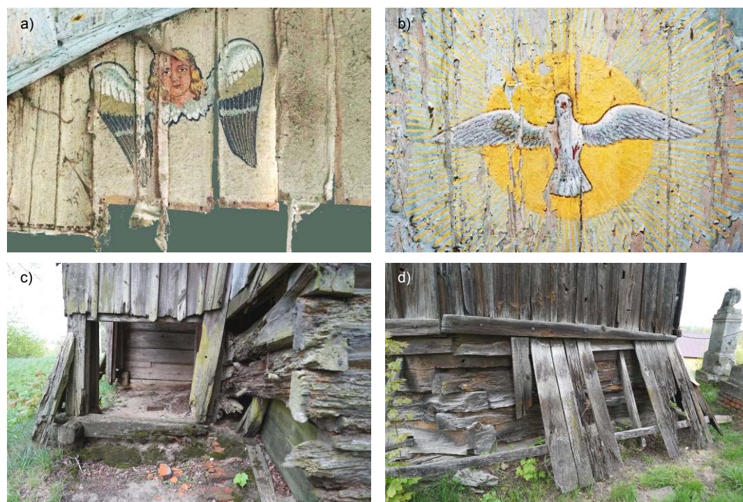
Fig. 8. Miękisz Stary, the condition of the wooden church in 2019: a) a fragment of the presbytery polychrome, b) a fragment of the presbytery polychrome, c) the basement destruction at the north porch, d) the presbytery destruction. Source: photo by author
