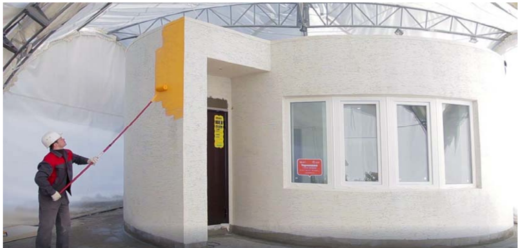
Fig. 16. Printing a house on a 3D printer. Stupino. Russia. Manufacturers: Apis Cor. Source: Fot. Apis Cor
