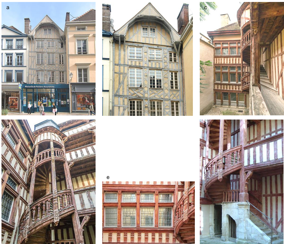
Fig. 13. Troyes, Hôtel du Lion - Renaissance façade and inner courtyard with a beautiful spiral staircase.
