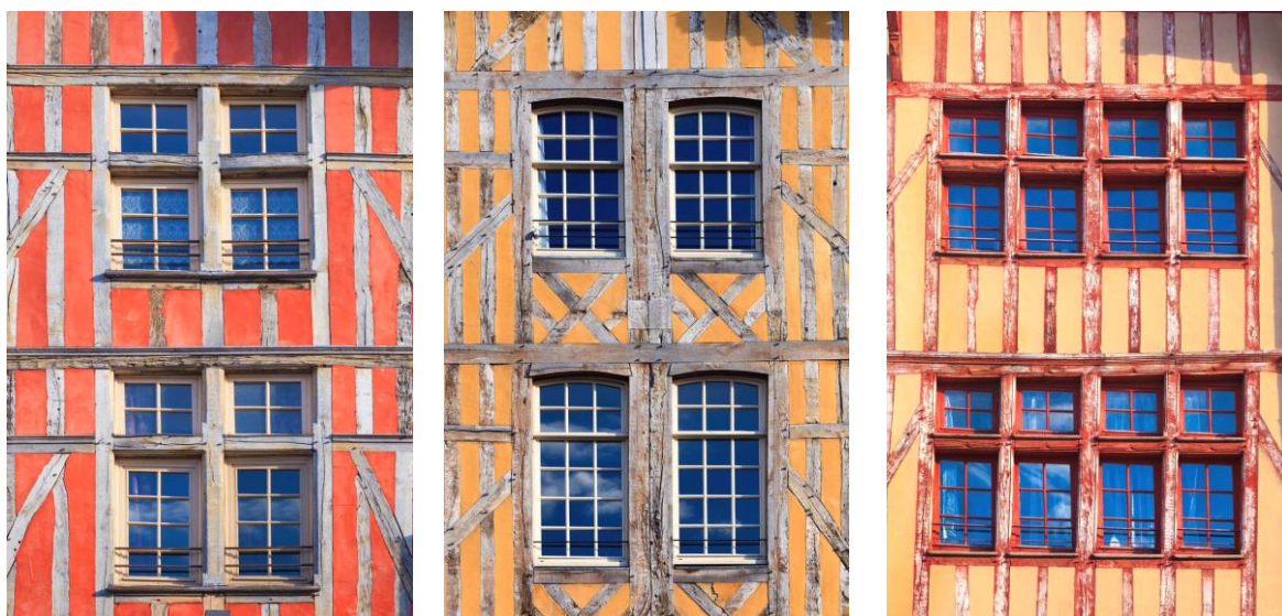
Fig. 8. Troyes, Examples of diversification of the "drawing" of the structure and colors of load-bearing walls of half-timbered houses. Source: Troyes rime
