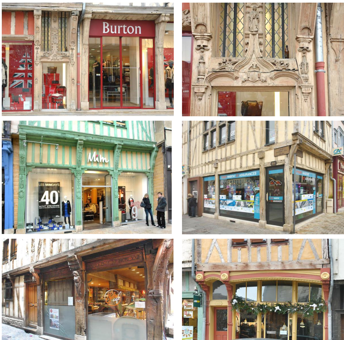
Fig. 16. Troyes, adapting the ground floors of half-timbered houses to modern commercial and gastronomic functions usually requires a significant "x-ray" - glazing of the filling between the wooden elements of the load-bearing frame.
