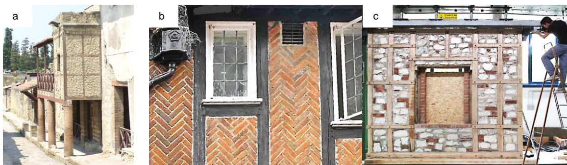
Fig. 5. Examples of filling the skeleton fields with stone or ceramics: a – Pompeii, b – Canterbury, c – Baraccata house, reconstruction.
