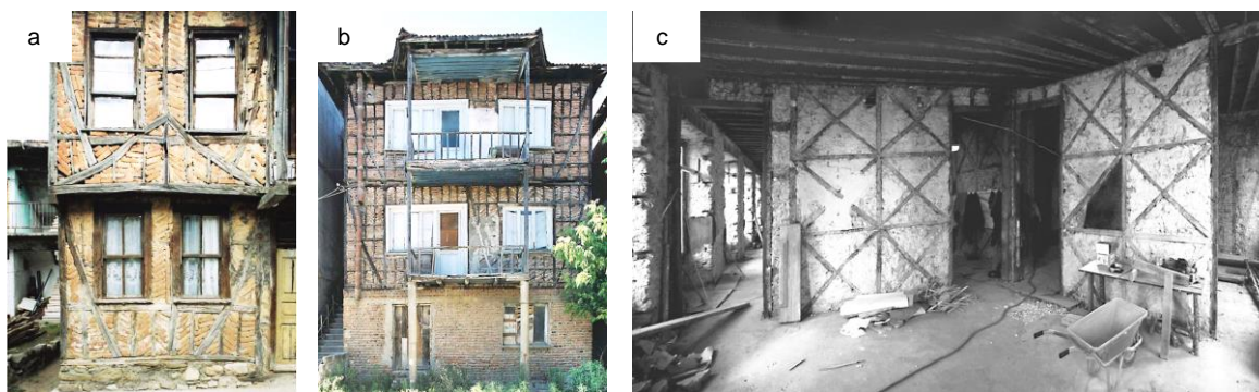
Fig. 6. The half-timbered stud wall shows better resistance to seismic shocks compared to massive masonry structures: a,b - Turkey, c - Lisbon.
