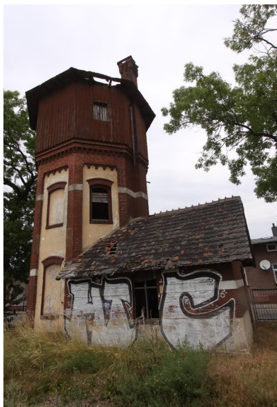
Fig. 2. Railway water tower, type R01, in Drawsko Pomorskie, with adjacent pump house, ©RB 2021.
