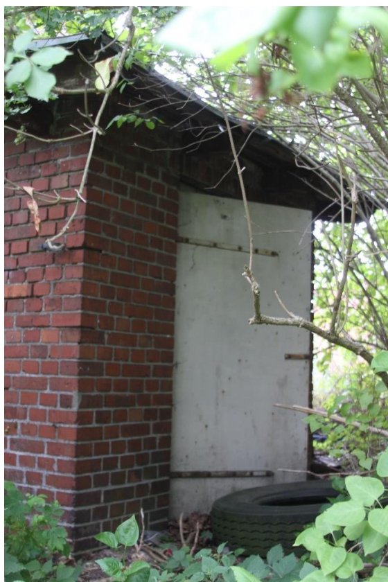
Fig. 1. Pump house adjacent to railway water tower in Śrem, type R05, ©RB 2021
