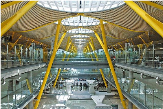
Fig. 14. Skylight and structure inside terminal Source: Adolfo Suárez, 2019
