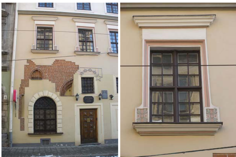
Fig. 2. Restoration of the renaissance façade polychromy with the sounding of gothic brick masonry (2, Ruska Str.) Source: photos by author
