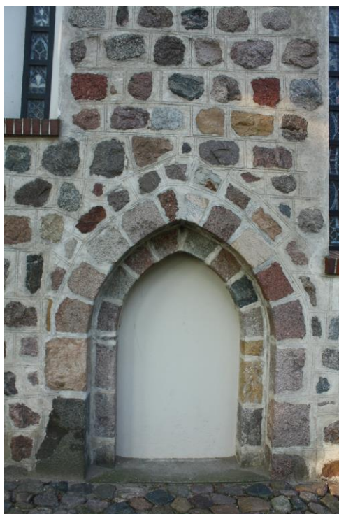
Fig. 3 Church in Mierzyn (Möringen) – ogival portal in the north wall; photo M.Plotkowiak
