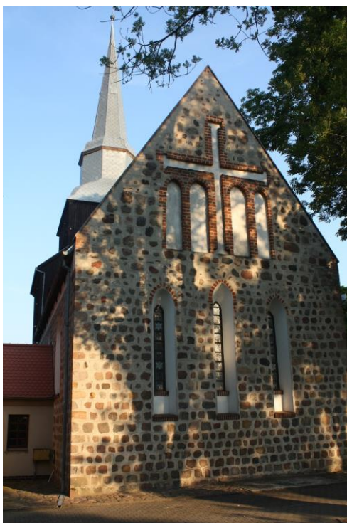
Fig. 2 Church in Mierzyn (Möringen) – view of the eastern gable wall; photo M.Plotkowiak
