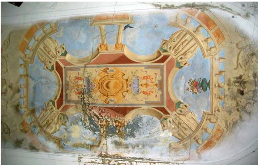
Fig. 15. Al secco mural of the upper store ceiling of the staircase in New Baroque Style ( di sotto in sù technique - open sky, illusive architecture, trompe-l'oeil technique) in 16 Verbytskyj Str. Source: photo by author
