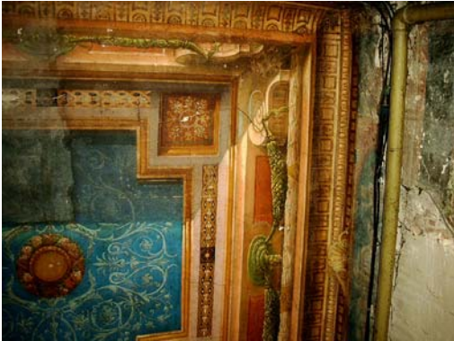
Fig. 14. Al secco painting in New Renaissance Style ( quadrature , turquoise background) on the ceiling of the staircase (9 Krakivska Str.). Source: photo by author
