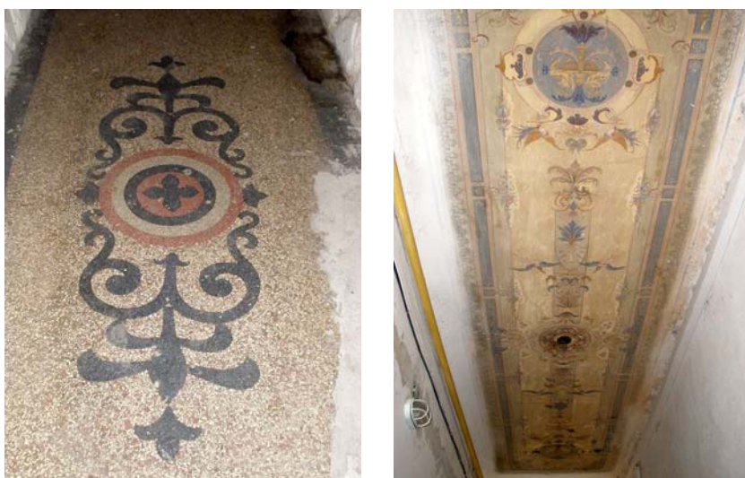
Fig. 44. Preserved elements of typical polychrome interior design of building in Historicism style: multicolored mural of the ceiling and tricolor terrazzo floor (7 Stavropihijaska Str.). Source: photo by author
