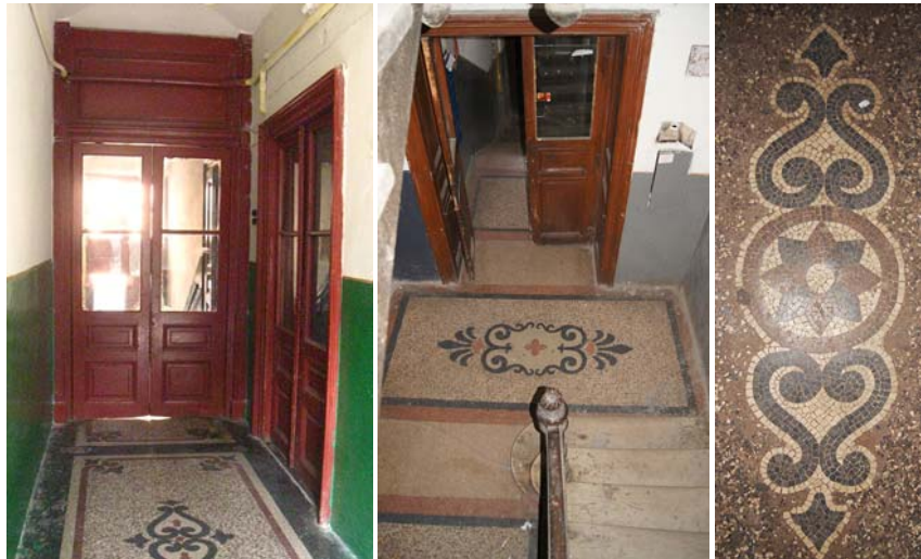
Fig. 32. Terrazzo floors in the interior spaces of buildings in the Historicism style (3 Romanchuka Str., 74 Franka Str., 65 Doroshenka Str.). Source: photo by author
