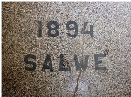
Fig. 29. Terrazzo floor with inscription of the erection of the building (40 Franka Str.). Source: photo by author
