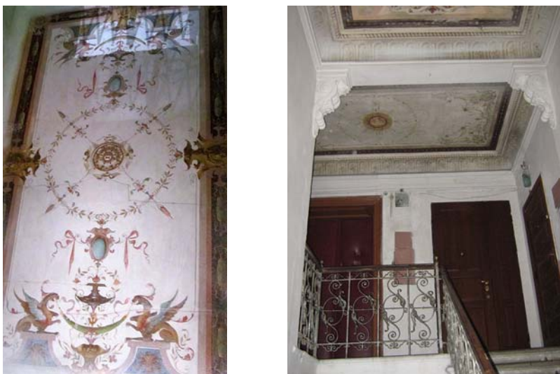
Fig. 12. Al secco paintings in New Renaissance Style (domination of light background) on the ceilings of the upper store of the staircase (48 Pekarska Str., 15 Hlibova Str.). Source: photos by author
