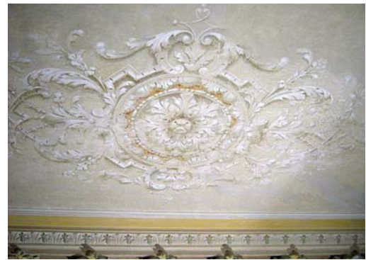
Fig. 5. The restored grisaille rosette (in Trompe-l'œil technique) on the vestibule ceiling (school in Konyshkoho Str.). Source: photo by author
