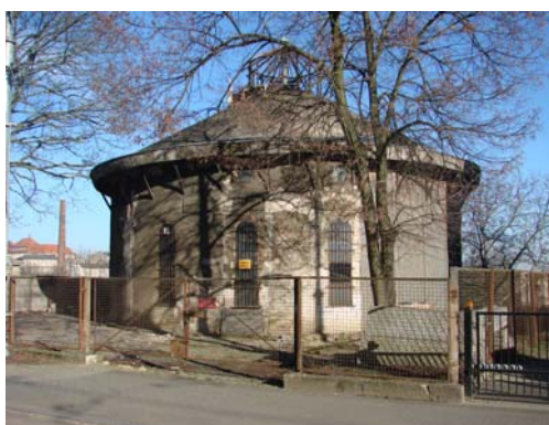
Fig. 2. View of a degraded water tower, 23.02.2019r. Source: author
