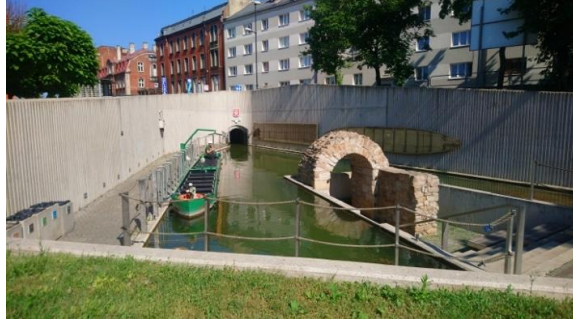
Fig. 16. The port at the Hereditary Adit on K. Miarki Street in its present state. Design: T. Konior Zabrze. Source: photo: T. Wagner 2019
