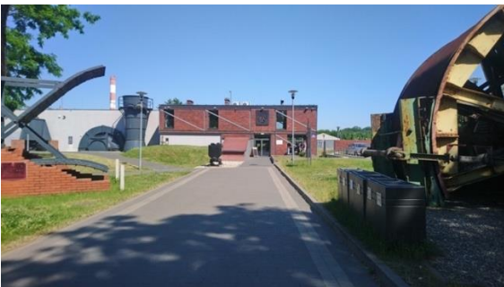
Fig. 17. Building of the entrance to the Królowa Luiza Adit - Sienkiewicza Street, Zabrze. Photo: T. Wagner 2019
