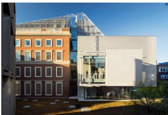
Fig. 13. View of the old and new parts of the museum and the passage connecting them. Source: Nic Lehoux
