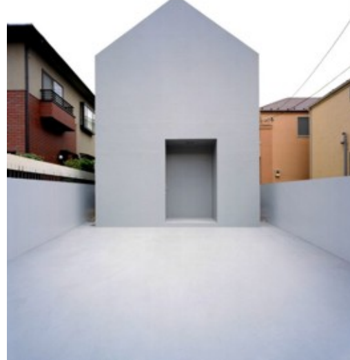
Ryc. 18. Ghost House , Datar, Sugunami, Tokio, Japonia, 2004-2006. Źródło: R. Gregory, Spirit levels: the Ghost House creates a haunting presence , The Architectural Review 12.2007
