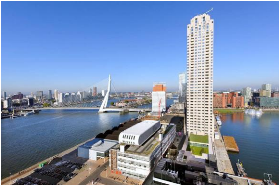
Fig. 4. High Residential Tall Building: New Orleans, Rotterdam, Netherlands. Architectural height: 158.4m, number of floors above: 46, number of apartments: 234; Author: Alvaro Siza. Source: Afasiaarchizine, 2010
