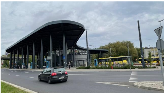
Fig. 13. Katowice Integrated Interchange System, Brynów Pętla Interchange, MERiTUM Projekt - the actual view of the facility, view from Kosciuszko Street. Source: photo M. Sroka-Bizoń
