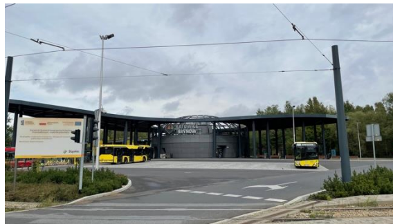
Fig. 14. Katowice Integrated Interchange System, Brynów Pętla Interchange, MERiTUM Projekt - actual view of the facility - the view from Rzepakowa Street. Source: photo M. Sroka-Bizoń
