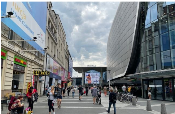
Fig. 11. New Katowice Railway Station with Galeria Katowicka, Neinver Polska - actual view of the public area in front of the railway station. Source: photo M. Sroka-Bizoń
