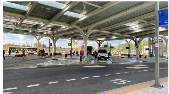
Fig. 18. Katowice Integrated Interchange System, Sądowa Interchange, MERITUM Projekt, the actual view of the facility - the view of the interior of the transportation space. Source: photo M. Sroka-Bizoń
