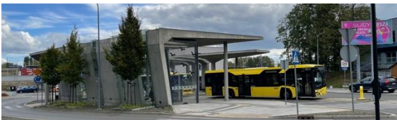
Fig. 15. Katowice Integrated Interchange System, Ligota Interchange, Grontmij Polska, actual view of the facility - the view from Panewnicka Street. Source: photo M. Sroka-Bizoń
