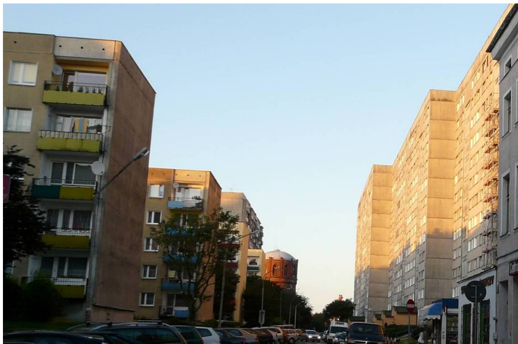
Fig. 2 Prefabricated slab houses in Kołobrzeg. Source: photograph by author.
