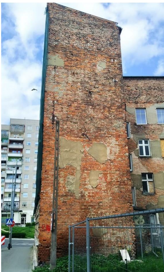
Fig. 6. Brick facade of the building. Source: Jarosław Piesik
