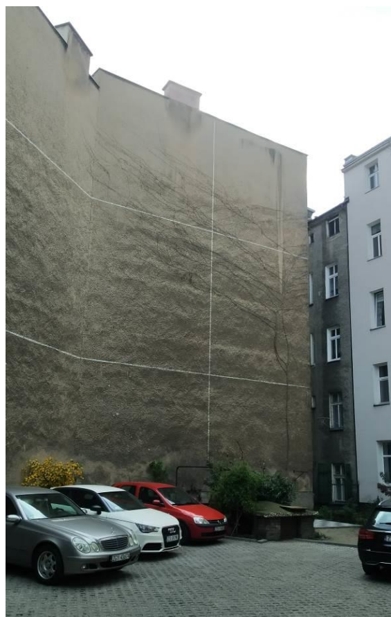
Fig. 5. The building's façade is covered with plaster. Source: Jarosław Piesik
