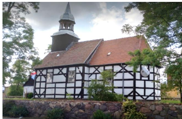
Fig. 4. Kalsko, church dedicated st. Bartholomew the Apostle from 1661 (mixed structure system - group 2). Source: autor's photo.
