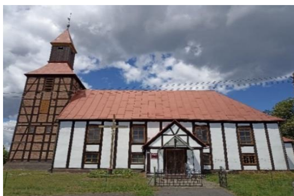
Fig. 8. Przynotecko, church of Our Lady of Częstochowa built from 1621 in half-timbered construction (group 3). Source: autor's photo.
