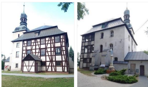
Fig. 11. Stare Drzewce, church of bl. Simon of Lipnica from 1599 in half-timbered construction and fragment of the walls made of white brick (group 3). Source: autor's photo.
