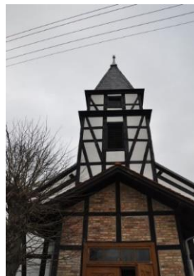
Fig. 10 a, b. Chartów, church of pw. Transfiguration of the Lord from 1828 in half-timbered construction (group 3). Source: autor's photo.
