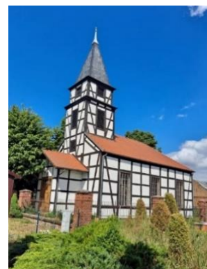
Fig. 10 a, b. Chartów, church of pw. Transfiguration of the Lord from 1828 in half-timbered construction (group 3). Source: autor's photo.
