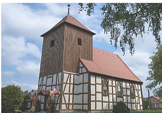
Fig. 7. Wysoka, church of st. Nicholas in half-timbered construction (group 3); from 1719 (tower) and 1730-1735 (nave body) Source: autor's photo.
