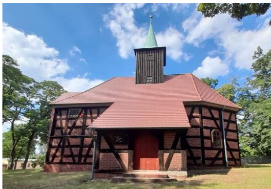
Fig. 9. Chocisz, church of Our Lady of Perpetual Help built from 1687 in half-timbered construction made of red brick (group 3). Source: autor's photo.
