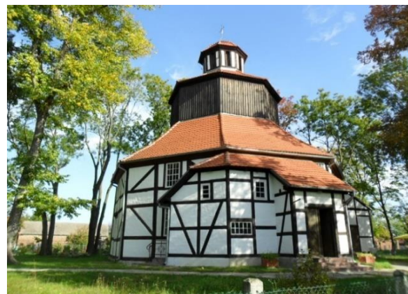
Fig. 6. Sękowice, church Holy Family in half-timbered construction, from 2nd half of the 17th century (group 3). Source: autor's photo.
