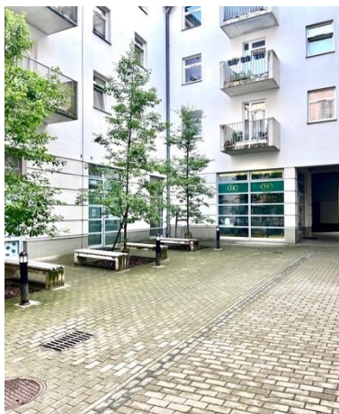
Fig. 4. Interior of quarter 23. Source: photo made by author, 2024
