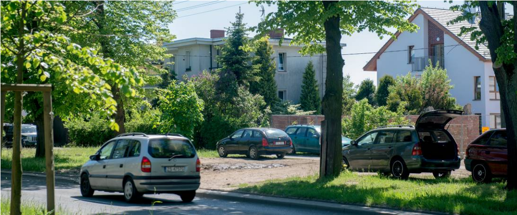
Fig. 3. Example of two post-war detached houses built on Szeroka street in Krzekowo. Source: photo by Waldemar Marzęcki
