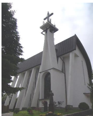
Fig. 4. B type church. Church of the Holiest Saviour in Rewal, architect Z. Abrahamowicz, 1976; photo D. Janisio-Pawłowska
