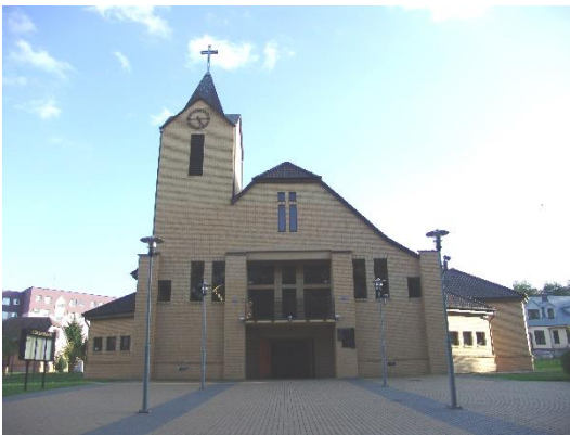
Fig. 11. A type church. Church of Christ the Good Shepherd in Szczecin, architect A. Zaniewska, 1998; photo: D. Janisio-Pawłowska
