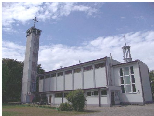
Fig. 9. E type church. Saint Michael the Archangel's Church in Wielgów, architect T. Szuta, W. Zięba, 1976; photo D. Janisio-Pawłowska
