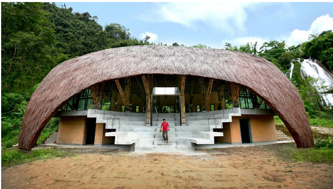
Fig. 5. 1+1>2 Architects, Chieng Yen Community House (2015) in Vietnam. Material solutions typical of Southeast Asia, Africa and South America. Combination of traditional local materials and construction techniques (structures made of wood, bamboo and reeds) with contemporary materials and construction technologies (reinforced concrete, ceramic brick). Original formal hybrids are produced as a result of these combinations. Source: Griffiths A. 2019
