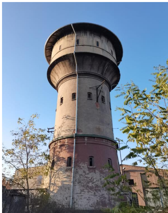
Fig. 4. Water tower No. 4 (at 2 Towarowa Street) in Kędzierzyn-Koźle. Source: ©WB 2022
