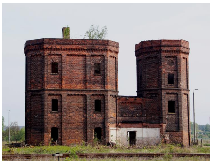
Fig. 7. Water tower No. 2 and 3 (single and double) in Kostrzyn nad Odrą. Source: ©WB 2022
