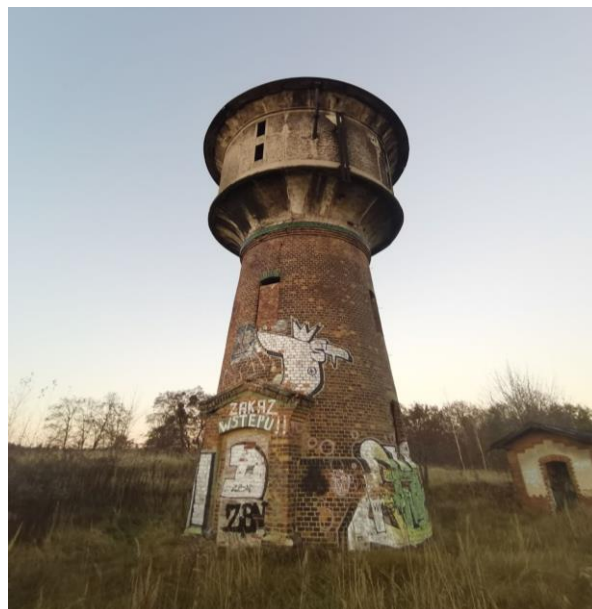
Fig. 5. Water tower No. 5 (in Kłodnica district) in Kędzierzyn-Koźle. Source: ©WB 2022
