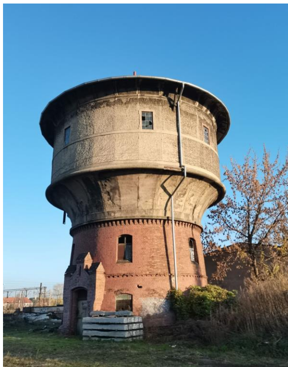
Fig. 3. Water tower No. 3 (at 12/14 Towarowa Street) in Kędzierzyn-Koźle. Source: ©WB 2022
