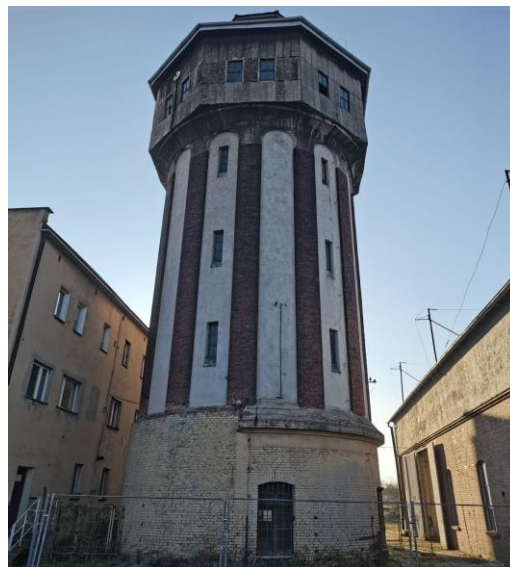
Fig. 2. Water tower No. 2 (at the locomotive depot) in Kędzierzyn-Koźle. Source: ©WB 2022
