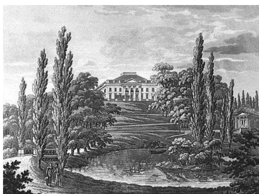
Fig. 1. Engraving. View of Belweder as viewed from Vistula river. Author F. Dietrich, 1827-1829. Source: [23]
