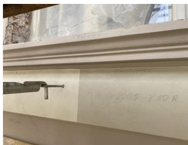
Fig. 3. Further color application trials prepared for evaluation by the heritage conservator. Source: by author
