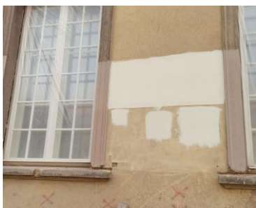
Fig. 4. Further color application trials prepared for evaluation by the heritage conservator. Source: by author
