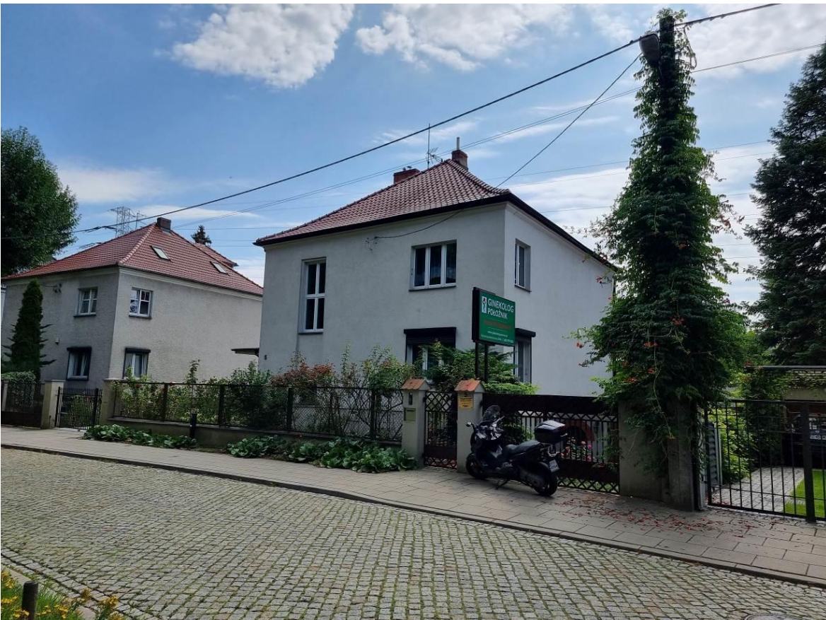
Fig. 17. Villas no 4 (to the left) and no 5 (center), Litewska st., Poznań (source: autor).
