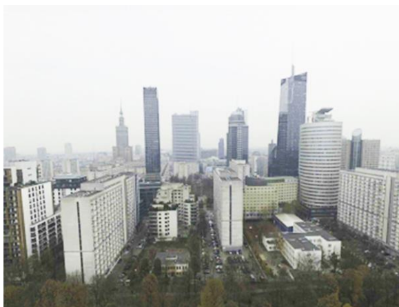
Fig 3 A fragment of downtown Warsaw - the existing state of spatial chaos; presentation of various buildings from various periods of the last 50 years. Source: photo from the drone Andrzej Grabski, 2018
