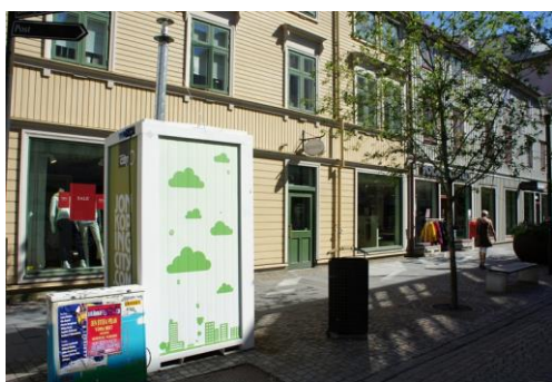
Fig. 13. Air pollution monitoring and treatment facility in Jönköping Centre. Source: author (2015)
