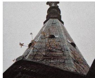
Fig. 9. Hollow welds in the tower's helmet. Source: Photo collections of Andrzej Rybarczyk and Mirosław Hamberg
