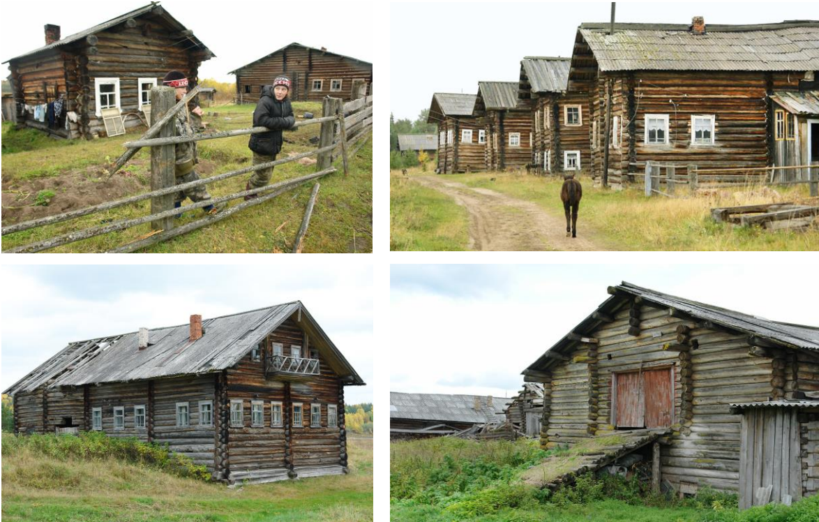
Fig. 12-15. The village of Kuczhas on the Pinega River, degradation of 120-year-old buildings. Permanently live here only two families... Source: photo author
