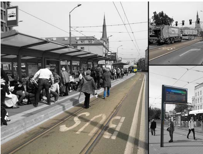
Fig. 1. Szczecin, integrated bus and tram stop at Brama Portowa; bus line at Brama Portowa; information board on the tram stop at Brama Portowa; Source: Olga Gazińska 16/05/2017
