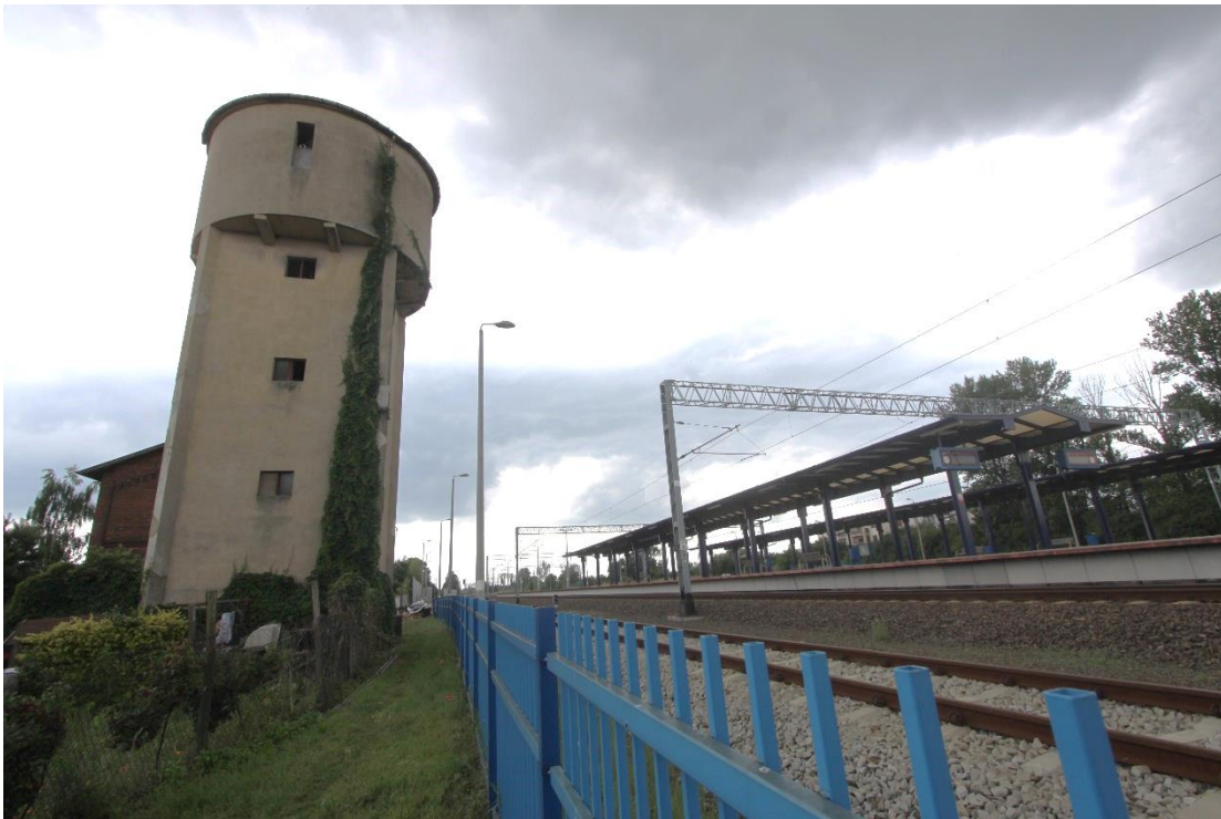
Fig. 15. Railway water tower in Czempin, type R25, ©RB 2021.
