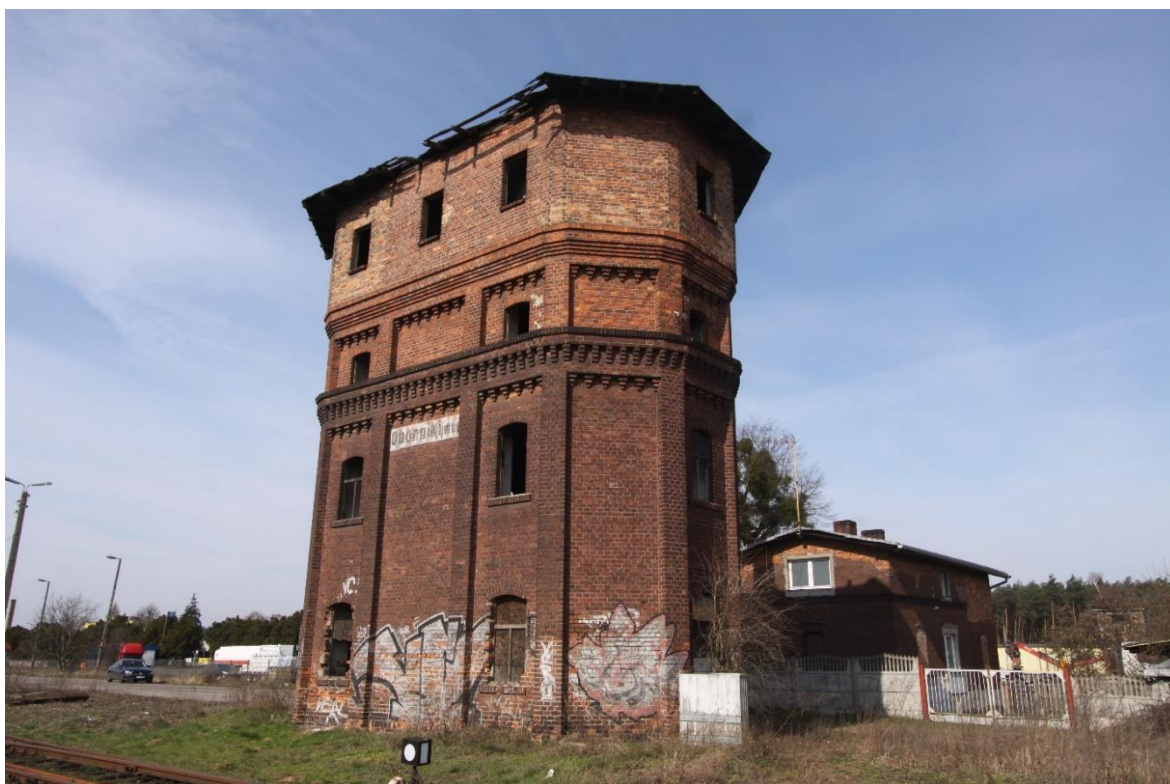
Fig. 3. Railway water tower in Oborniki, type R02, ©RB 2021.
