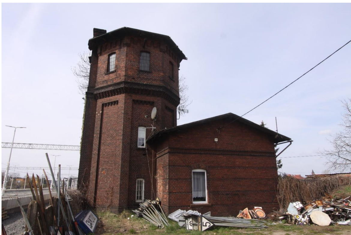
Fig. 2. Railway water tower in Wronki, type R01, ©RB 2021.
