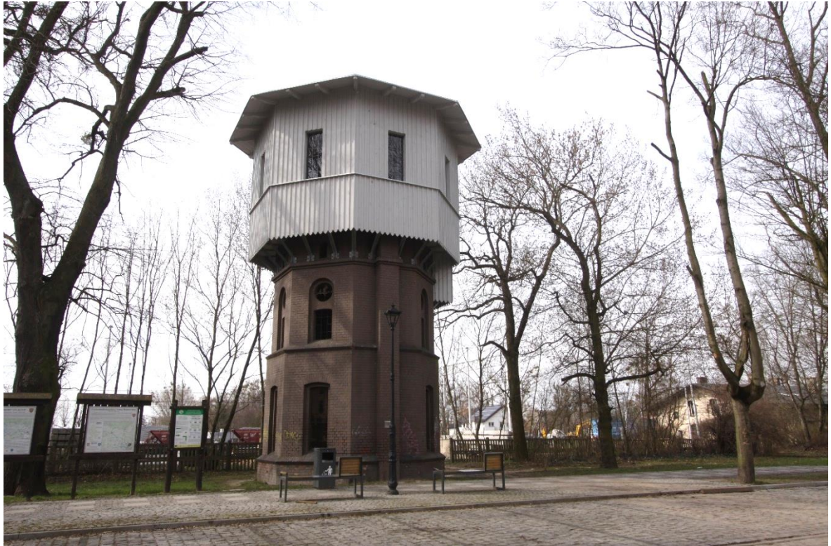
Fig. 4. Railway water tower in Szamotuły, type R03, ©RB 2021.
