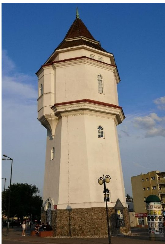
Fig. 12. Railway water tower in Konin, type R15, ©RB 2021.
