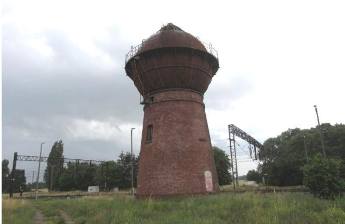
Fig. 9. Railway water tower in Runowo Pomorskie, type R08, ©RB 2021.
