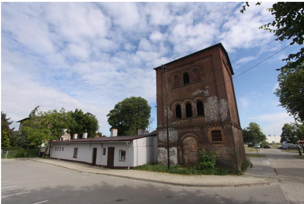
Fig. 5. Railway water tower in Pobiedziska, type R04B, ©RB 2021.
