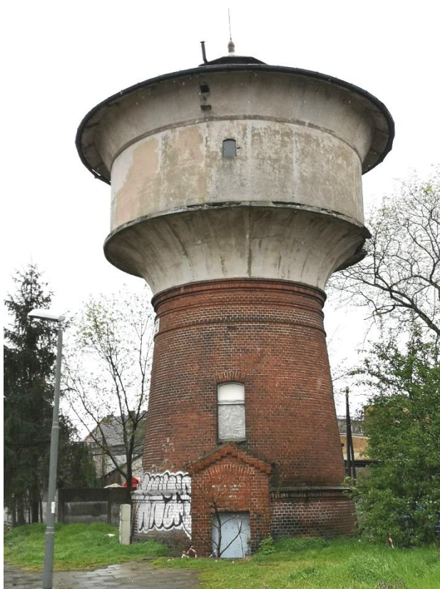
Fig. 7. Railway water tower in Międzyrzecz, type R05, ©RB 2021.
