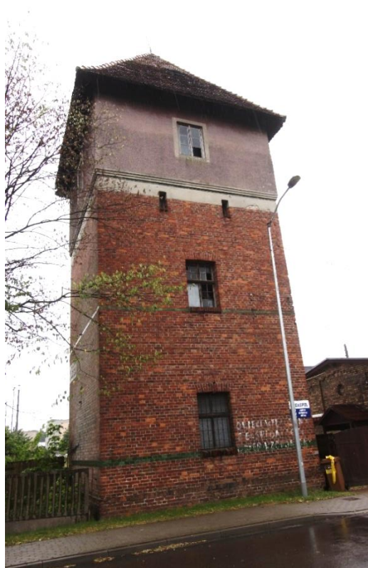
Fig. 13. Railway water tower in Łobez, type R18, ©RB 2021.
