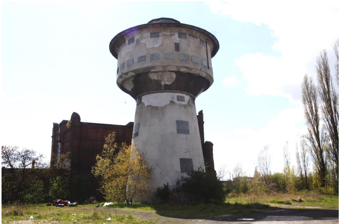
Fig. 8. Railway water tower in Poznań with high capacity water tank, type R05, ©RB 2021.
