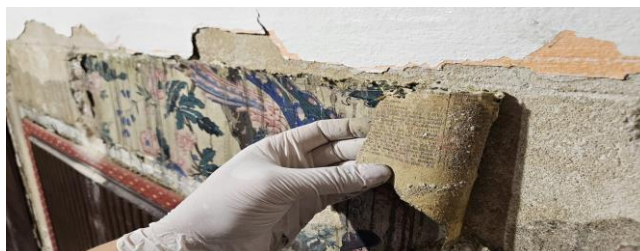
Fig. 9. Original wall covering of one of the studies on the first floor of the building, photo from restoration work. Source: photo provided by the Pszczyna Castle Museum.
