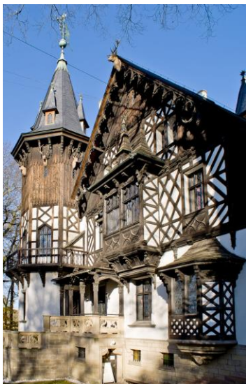
Fig. 5. Western facade. Photo showing the complexity of the future renovation and restoration work – stone, plaster and wood patterns. Source: photo by the author 2022.
