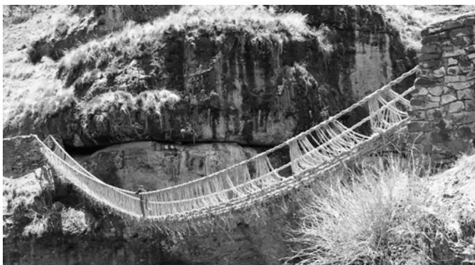
Fig. 2. Keshwa Chaca – suspension bridge in the Andes, rebuilt by the local community with the use of techniques applied in the past. Source: [11]
