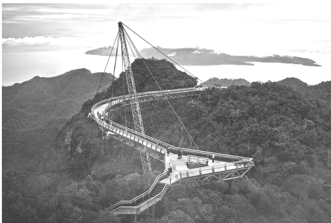
Fig. 11. Cable-stayed structure of Langkawi Sky Bridge. Source: [29]
