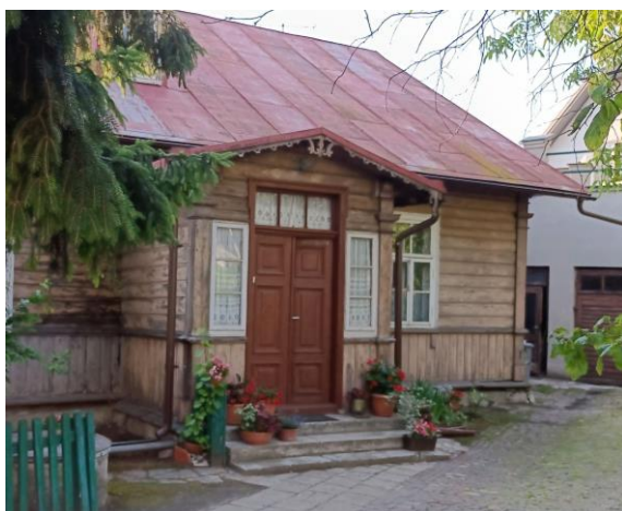
Fig. 1. The photos illustrate a building at 2 Narutowicza Street in Hrubieszow, an example of preserving the original window woodwork with a narrow profile forming a division. Source: author
