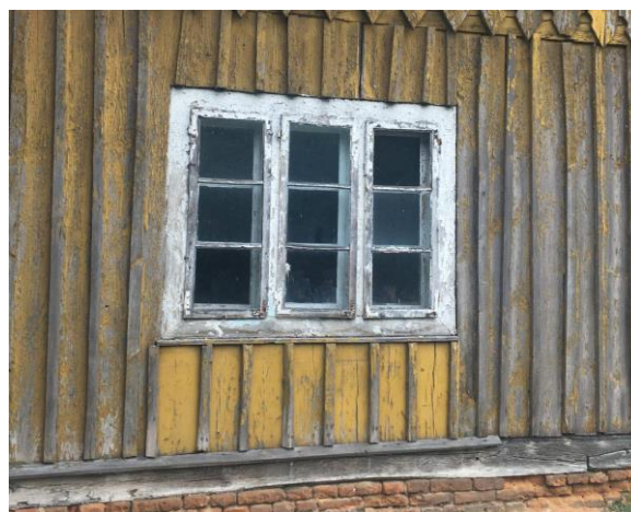
Fig. 2. The old paint should be removed wet with sharp hands. The wood receives an intact and opaque fresh coat of linoleum paint. Source: author
