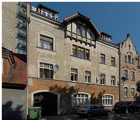
Fig. 14b. Zielona Góra. A residential building in the frontage layout at the Bolesława Chrobrego 38 Street. Wooden design was made in the skeleton technique and plastered on the gable ledge. Source: autor's photo
