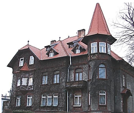
Fig. 13. Zielona Góra. „House with a tower” with an attic and the tower made of a half-timbered structure at 7 Batrosza Głowackiego Street. Source: autor's photo.
