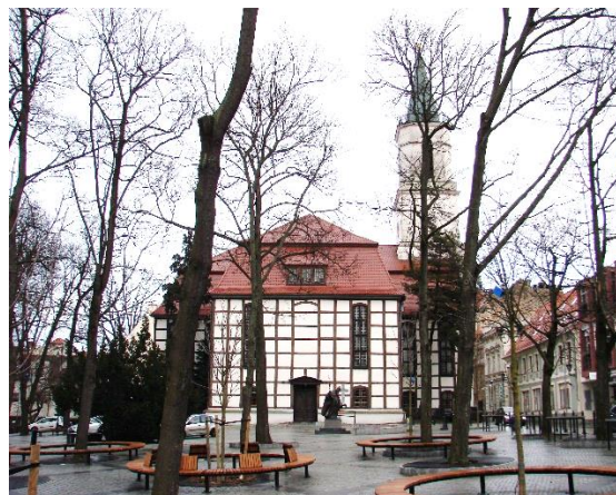
Fig. 2c. Zielona Góra, the Old Town. View of the body of the post-Evangelical church built in a half-timbered structure (1746-1748) with a later tower from 1828. Today - the Catholic Church of Our Lady of Częstochowa. Source: autor's photo
