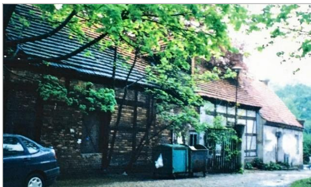
Fig. 15. Zielona Góra. Two farm buildings at the 17 Wrocławska Street: on the left and middle – built was in the "half-timbered" technique; on the right – a residential building was built in the traditional technique. Source: autor's photo
