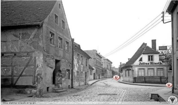
Fig. 3. Zielona Góra. A residential building erected in a gable layout at 43 Wrocławska Street, made of half-timbered technology, plastered. Source: Mia. 2014
