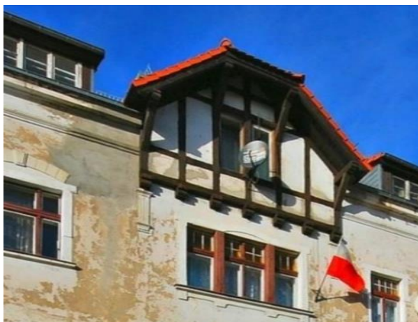
Fig. 14a. Zielona Góra. A residential building in the frontage layout at the Bolesława Chrobrego 38 Street. Wooden design was made in the skeleton technique and plastered on the gable ledge. Source: autor's photo
