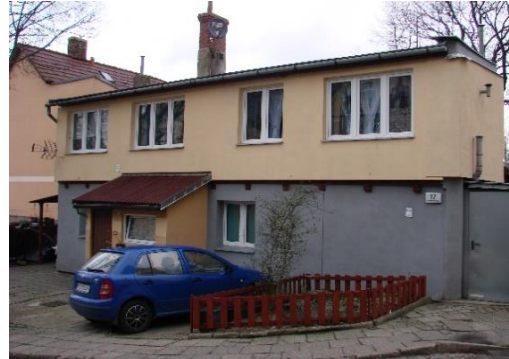
Fig. 4. Zielona Góra. A residential building made out of half-timbered structure at 17 Krzywoustego Street. Source: autor's photo
