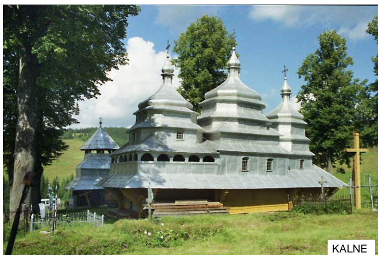
Fig. 40,41. Examples of wooden Orthodox churches in Ukraine covered with sheet metal. This covering, while protecting from precipitation, at the same time increases the moisture content of the wooden supporting structure. Source: author's photographs (1996)
