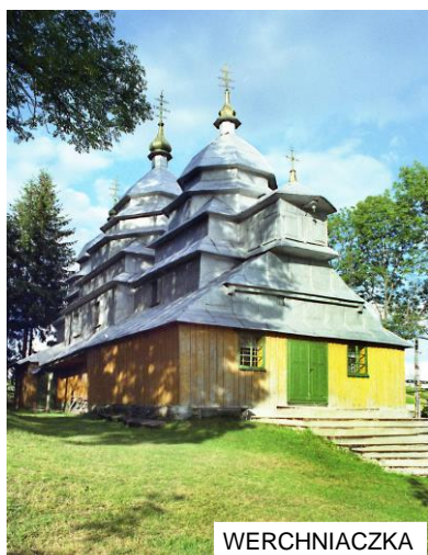
Fig. 40,41. Examples of wooden Orthodox churches in Ukraine covered with sheet metal. This covering, while protecting from precipitation, at the same time increases the moisture content of the wooden supporting structure. Source: author's photographs (1996)
