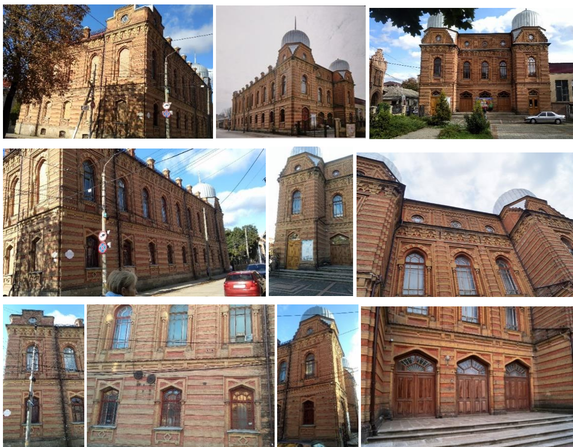
Fig. 7. Facades and a fragment of the facade of the Elisavetgrad Choral Synagogue. Source: T.Penyaz's photo;
