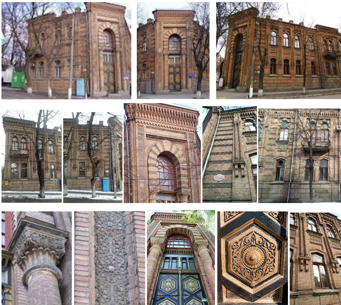
Fig. 6. Facades of I. Goldenberg water clinic. Source: T. Penyaz's photo
