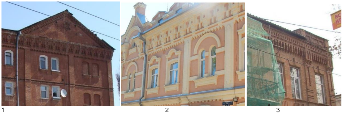
Fig. 8. Decoration of frieze and cornice elements, that repeated in the architecture of other buildings of Kropyvnytskyi: Of the choral Synagogue - 1. Hoholya str. 44; 2. Shulgyinikh str. 32; Of the I. A. Goldenberg's water clinic - 3. T. Karpy str., 55; Source: T. Penyaz's photo;
