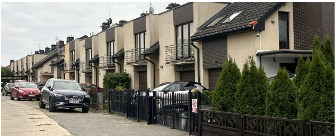
Fig. 6. Photographic documentation illustrating the issue depicted in the diagram (Fig. 5). Source: Author's own photographs, 2024.
