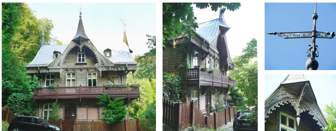
Fig. 11, 12, 13, 14. Gdańsk-Wrzeszcz (Danzig-Langführ), building and detail of the former forester's lodge ( Forsthaus ). Source: original photos 2020
