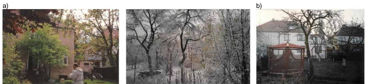
Fig. 19. Picture "a": The house from the garden side (north) before 1995. Picture "b" from the year 2001. Source: Authors' photographs
