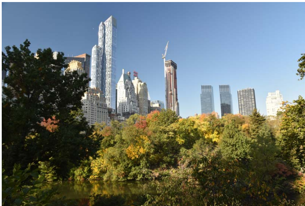
Fig. 7. Southern frontage of the building development along Central Park. In the foreground: One57 (Christian de Portzamparc, 2014). In the background: the construction of 220 Central Park South (Robert A.M. Stern); author's photograph
