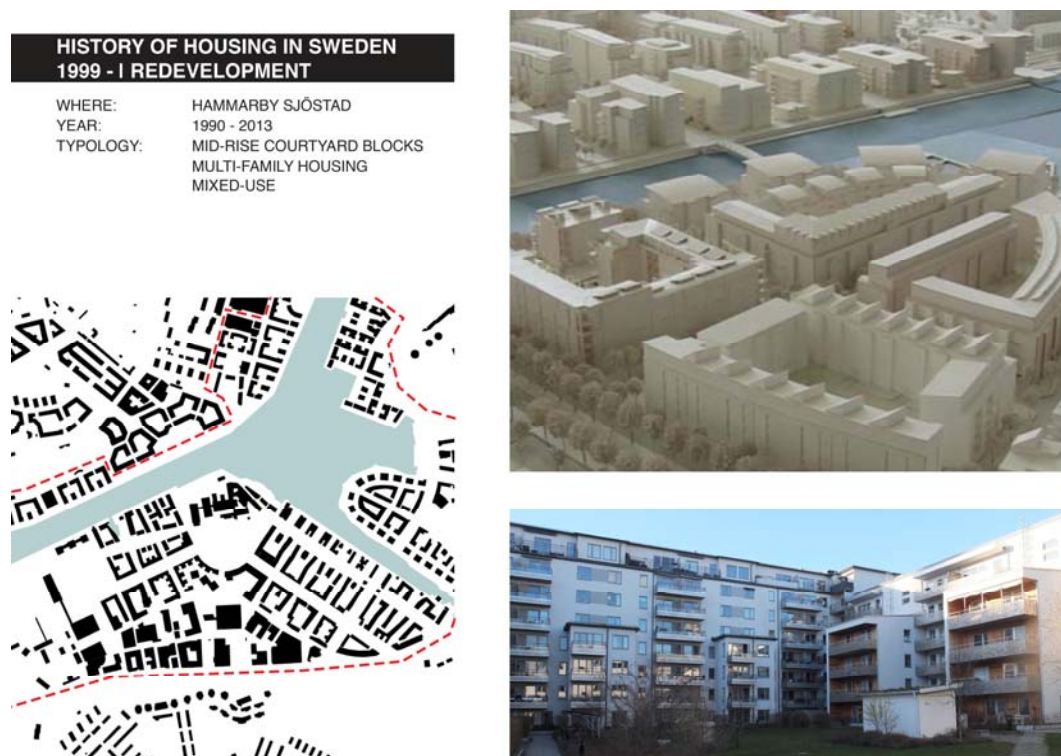
Fig. 12. Housing estate Hammarby Sjöstad, 1990-2013. Source: a) Authors, b) Mock-up, consulting company SWECO 2014 [14], c) K. Urbanowicz
