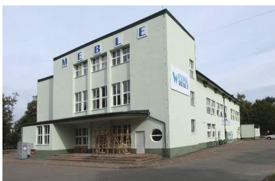
Fig. 12. The Forester's House. View from the south-west. Photo 2024. Photo 2024. Source: author.
