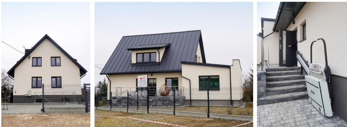
Fig. 3. Building in Biała Podlaska after modernization and adaptation to the function of a family care home.
