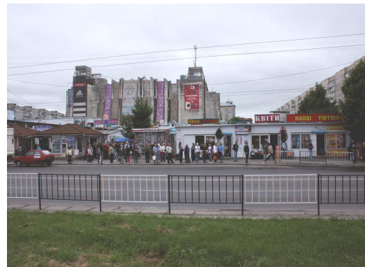
Fig. 3. New central department store in Lviv and neighboring territories (2013 year). Viewpoint №2. Source: A.Hoblyk
