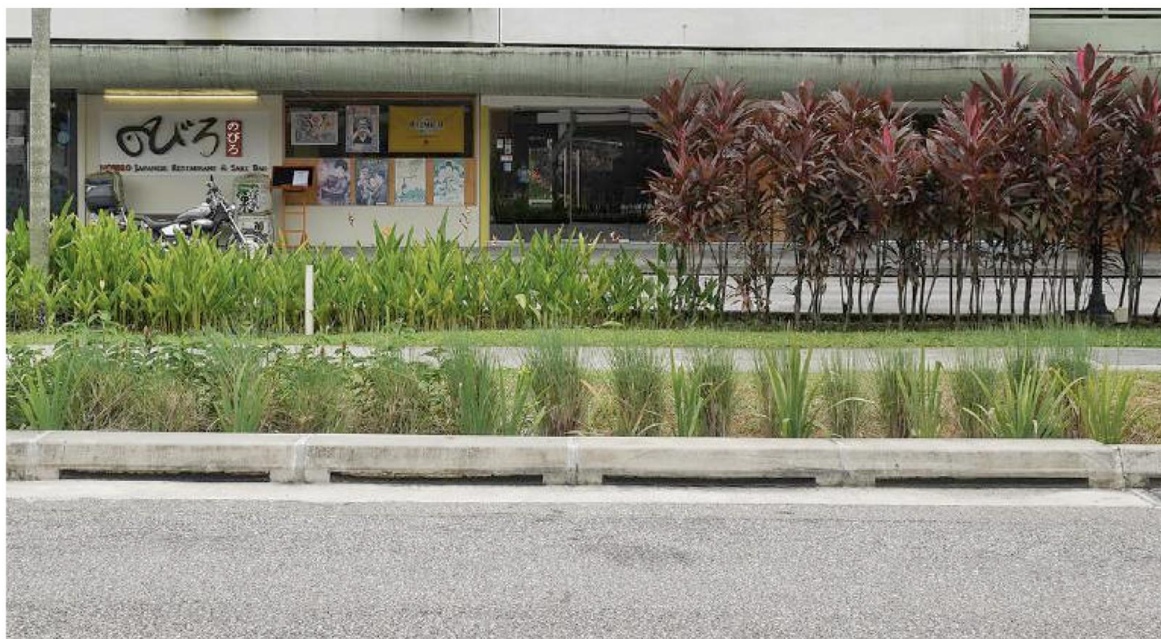
Fig. 2. Example of an in-street bioretention system (Faber Hill estate) ABC Waters Design Features. Source: Condensed, 2018a, p. 33 Chapter 7.
