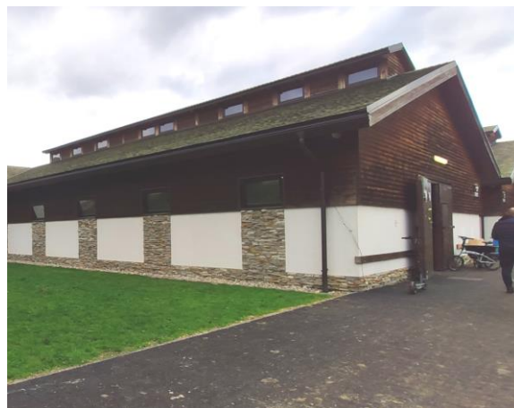
Fig. 3. Finishing the façade of a stable of natural stone and wood. Source: photo author
