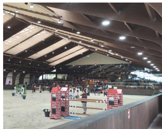
Fig. 5. Riding hall – internal view. Source: photo author.
