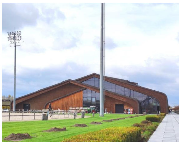
Fig. 4. Riding hall – external view. Source: photo author
