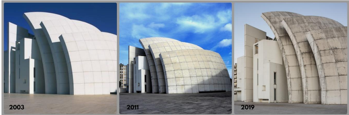
Fig. 3. Degradation of \text{TiO}_2 performance as a component of surface paints. Chiesa di Dio Padre Misericordioso, arch. Richard Meier. Source: by authors
