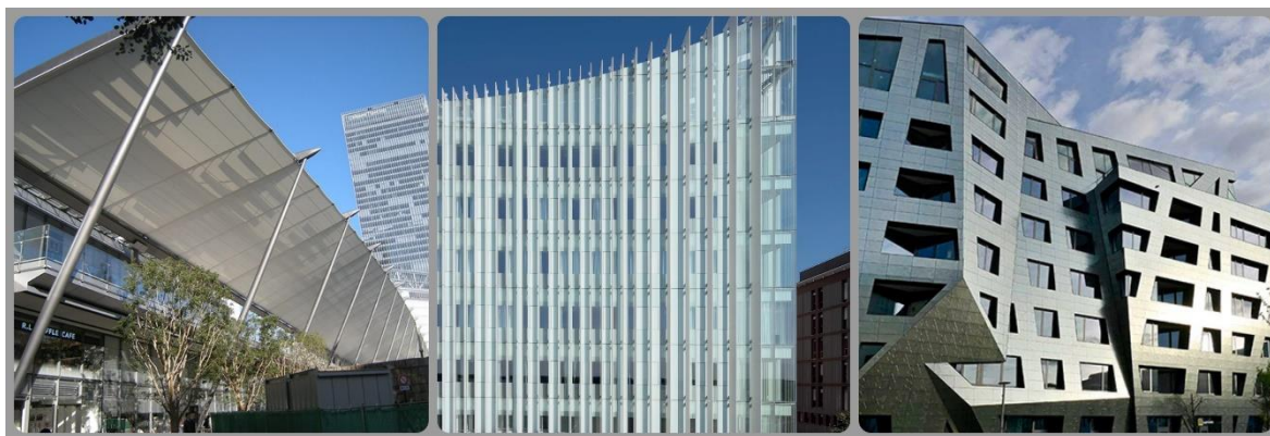
Fig.7. Different materials including \text{TiO}_2 photocatalyst. Left: Tokio Grand Station roof. Middle: San Raffaele Hospital in Milan. Right: Casalgrande Padana in Berlin. Source: by authors.
